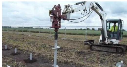
Fig 1. Screw piles being installed.
